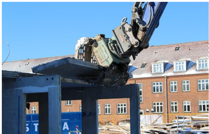
Figure 8 Dismantling of concrete element for re-use (Source: Danish Technological Institute)
